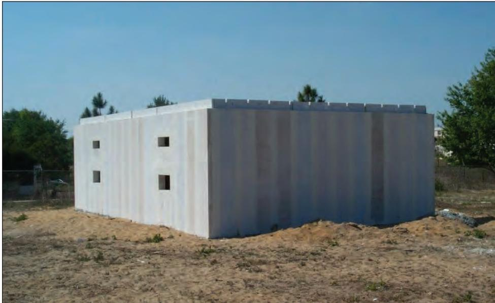
This 900 square foot communication equipment building shell made of AERCON wall and roof panels was built from start to finish in 8 hours.
